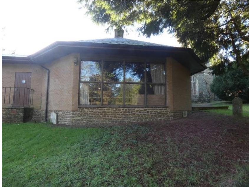
North elevation of Chapter House
